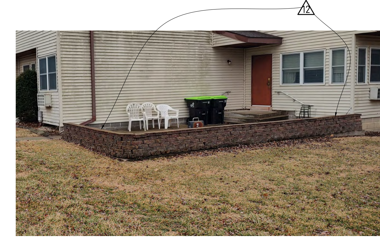
2 EXISTING MODULAR RETAINING WALL IL-71-13/PITTSFIELD
