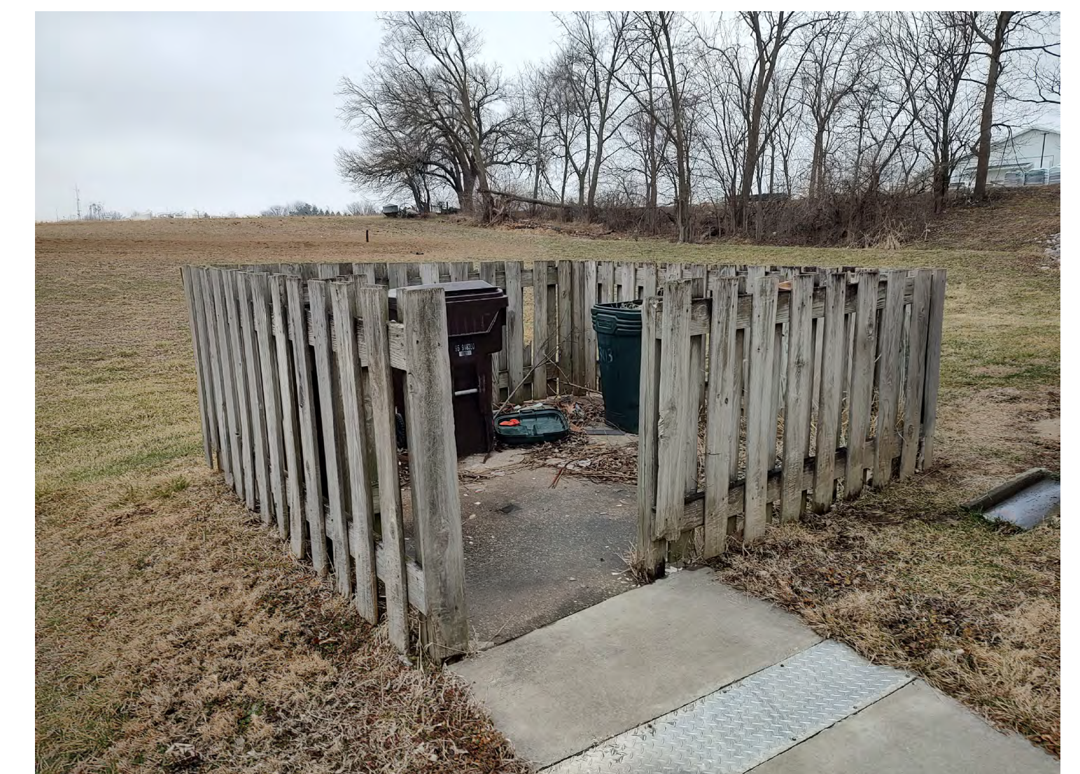
2 EXISTING TRASH SCREEN C-2 IL-71-9/PITTSFIELD
